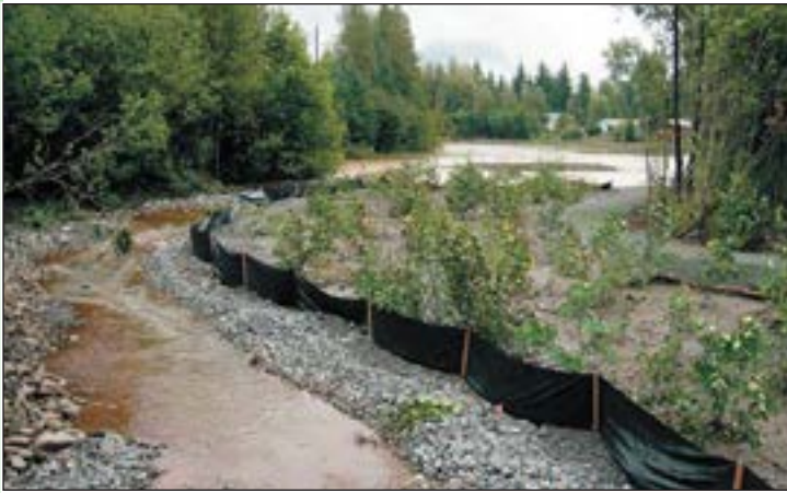
Alders transplanted along stream channel - 2006
