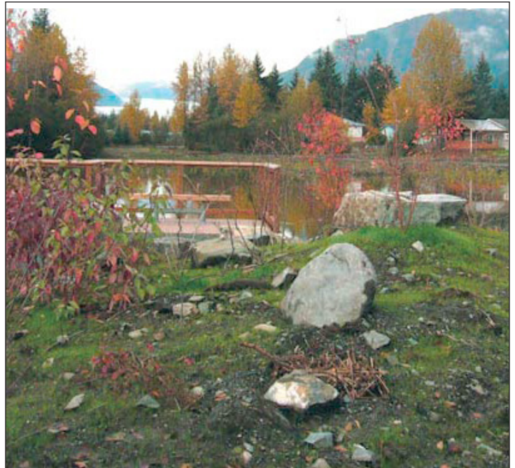
Finished observation deck & gathering area - 2006
